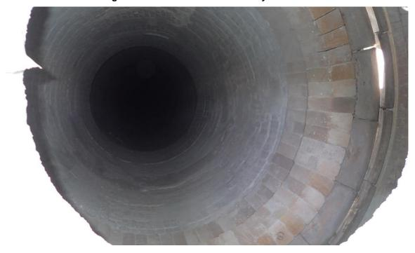
Figure 12-17 New fireproof lining at the end of the 80 m tube
