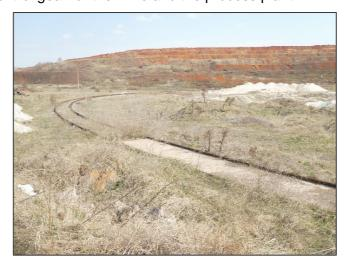
Figure 13-1 Existing rail track - partly interrupted and not maintained
