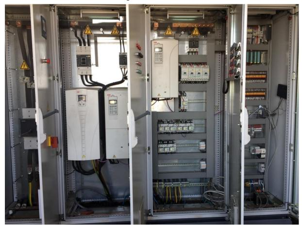
Figure 12-19 Control cabinet for rotary kiln
