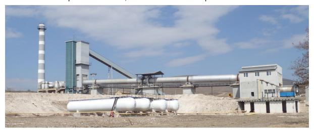
Figure 12-15 Rotary kiln during site visit in March 2019, in front the new gas tanks (Propane 70% and Butane 30%)
